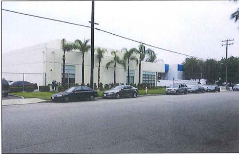
View looking northeast towards the business located adjacent to the project site.
