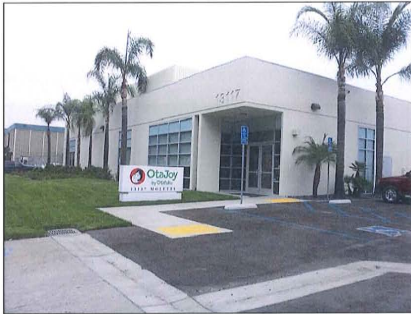
View looking towards the main public entrance to the Otafuko Foods plant. No modifications will be made to this building.
