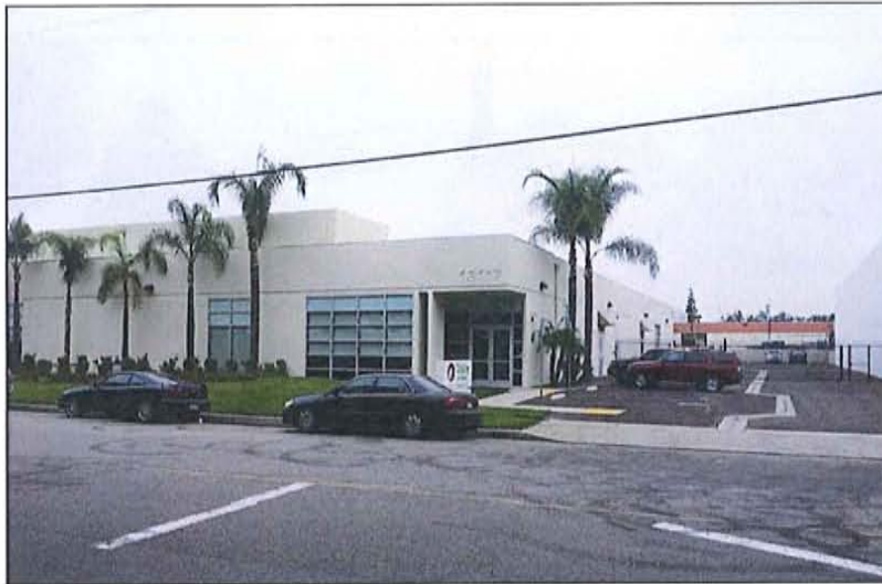
View looking across Molette Street towards the Otafuko plant.
